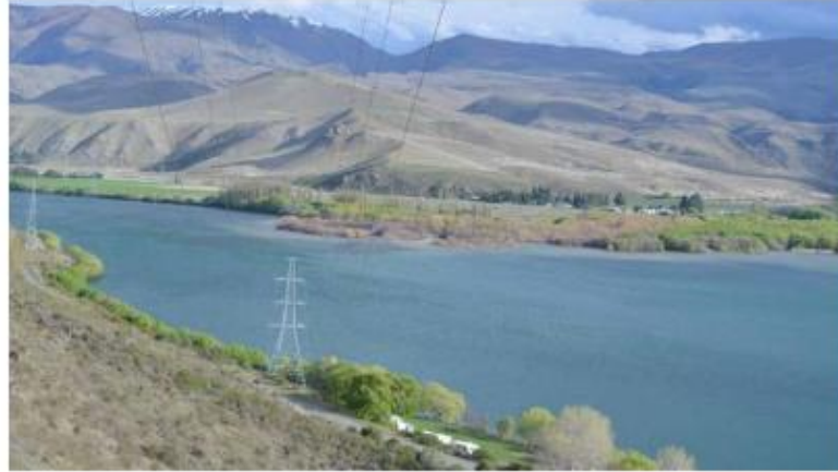
Transmission lines near Transpower's Benmore substation.
